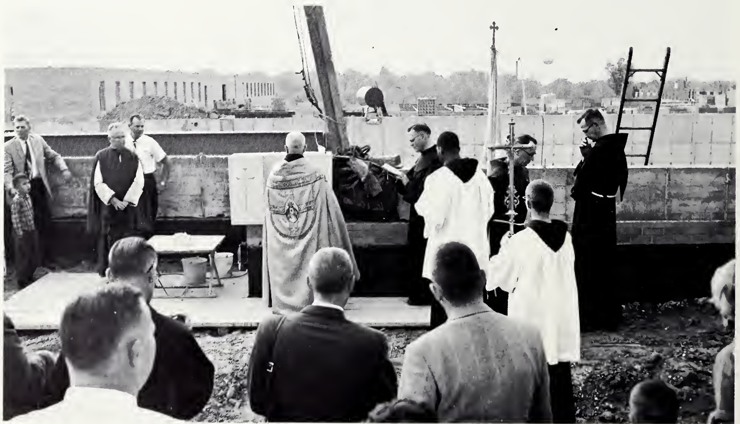
The Very Rev. Dominic Limacher, O.F.M., Minister Provincial, offered prayers at the corner stone laying of the new Seminary. Incompleted buildings may be seen in the background. Occupancy
